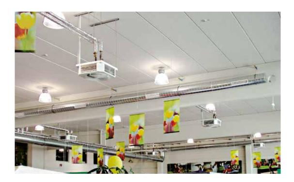
The **Elegant ECM** series uses an innovative brushless synchronous permanent magnet electric motor controlled by an inverter card that is directly installed on the unit.
