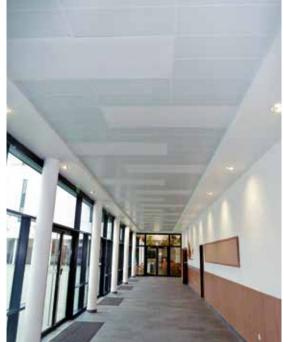
thick) protected by an aluminium sheet (25 micron thick) to be mounted on the top of the panel.The insulation is in Class A1 according to EN 13501-1 standard.
