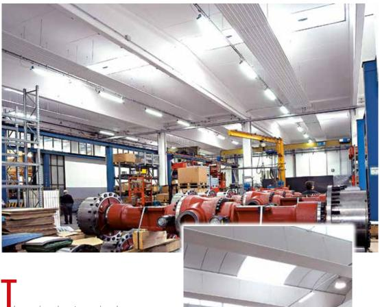
he main advantages involve exceptionally uniform temperature in the environment, fast stabilisation of the operating conditions, and a particularly simple and long lasting system with reduced energy consumption (almost no power consumption).
